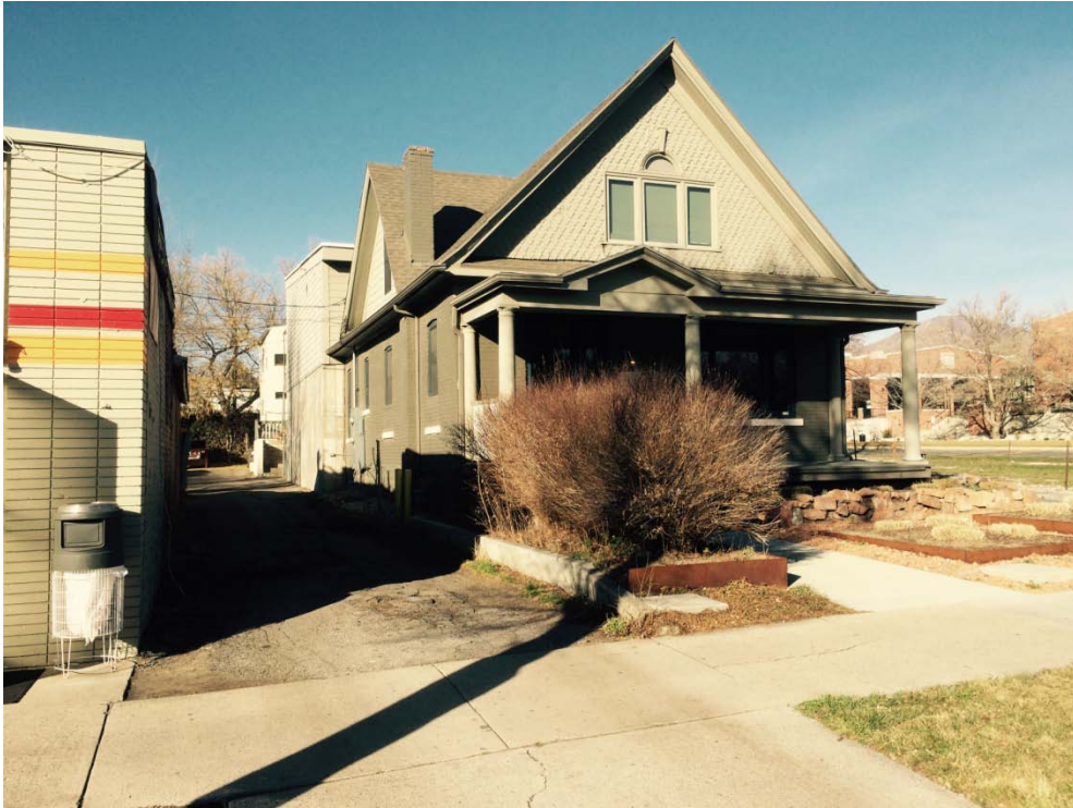
Neighboring commercial building east of the subject parcels
