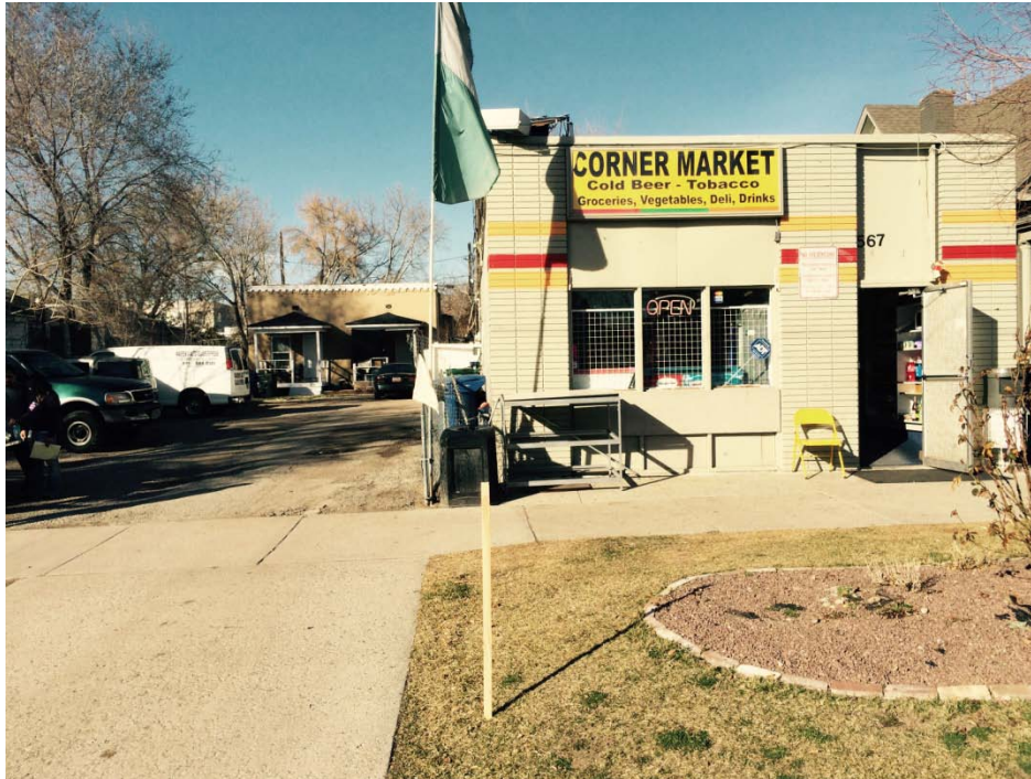
Existing contributing duplex with parking lot (left) and retail store (right)
